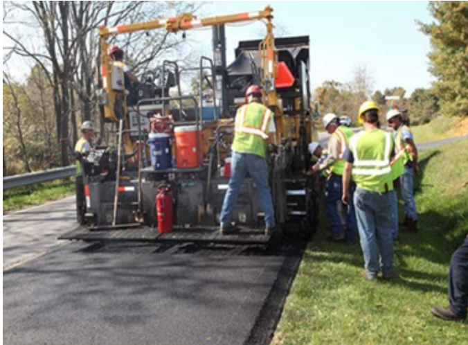
Roadway shoulder paved with a shoulder wedge.
